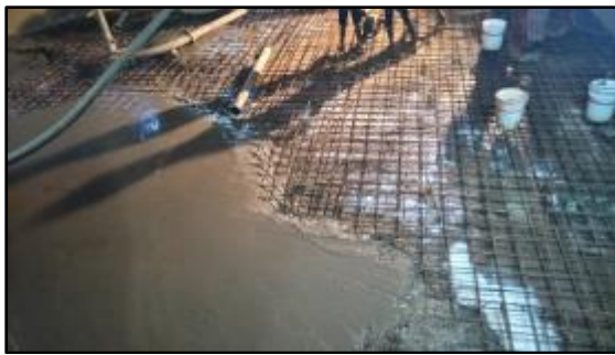
Fig.31 Spreading of Armorcrete chemical on the existing raft slab
