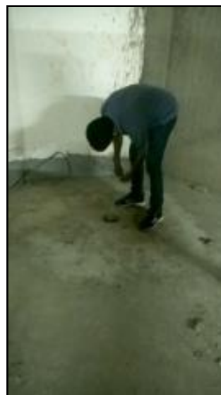
Fig.8 Checking the Depth of Anchor pile
