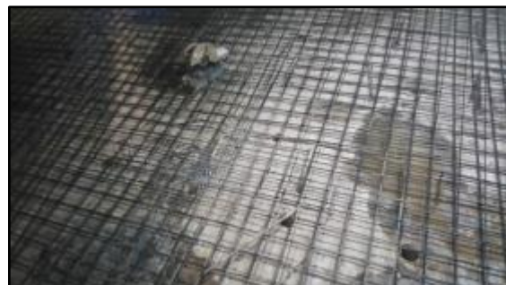
Fig.28 Full completion of laying of top steel
