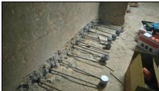
Fig.24 Fixing the bar in the drilled hole (Anchor Resin)
