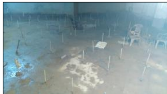
Fig.21 Cleaning of basement and completion of all the anchor piles
