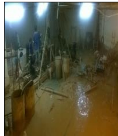
Fig.15 During the pressurized grouting in progress
