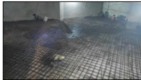
Fig.27 Laying of top steel
