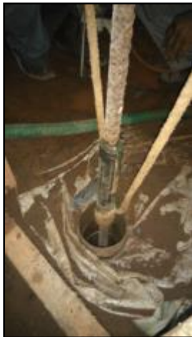
Fig.11 Insertion/placing of bar in the bore hole
