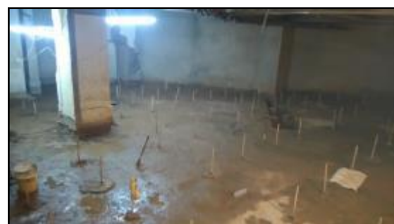
Fig.22 Final view of completion of anchor piles
