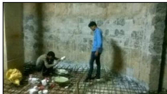
Fig.29 Before the commencement of concreting application of NITOBOND to the existing raft slab
