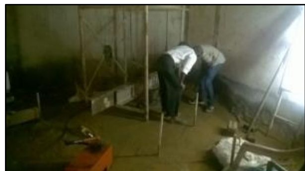
Fig.35 Documentation of dial gauge readings for load tests on piles
