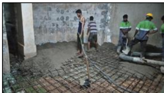
Fig.30 Concreting work in progress for new raft slab
