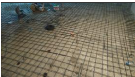
Fig.26 Bending the anchor pile steel in the new raft
