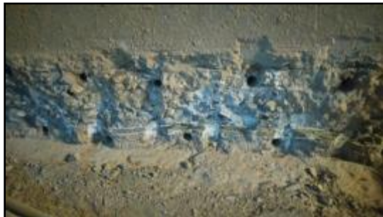
Fig.23 Drilling and cleaning the hole
