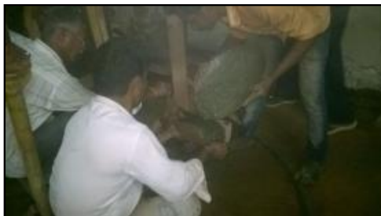
Fig.18 Pouring the concrete in the bore hole
