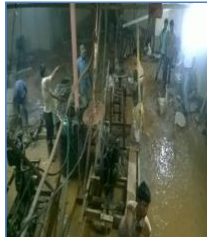
Fig.14 Plugging the anchor pile and starting the grouting process
