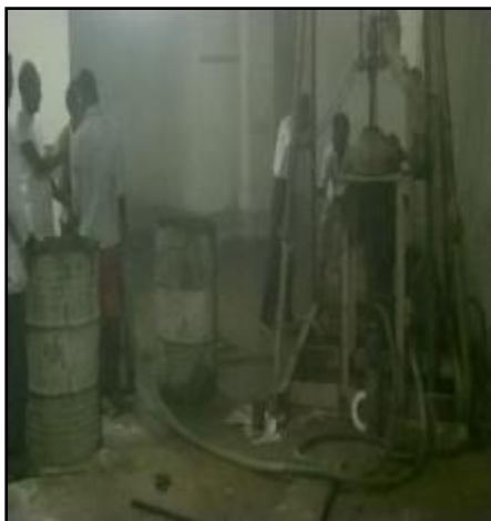
Fig.12 Preparing the proportion of 1:6 for grouting
