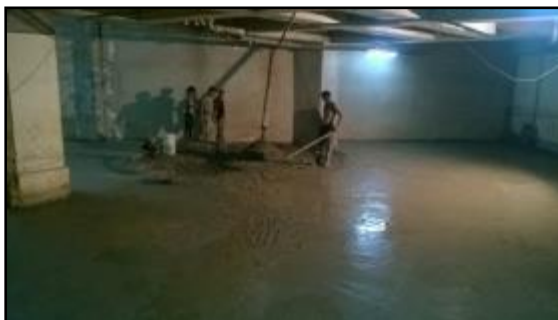
Fig.32 Final view after concreting of the new raft slab
