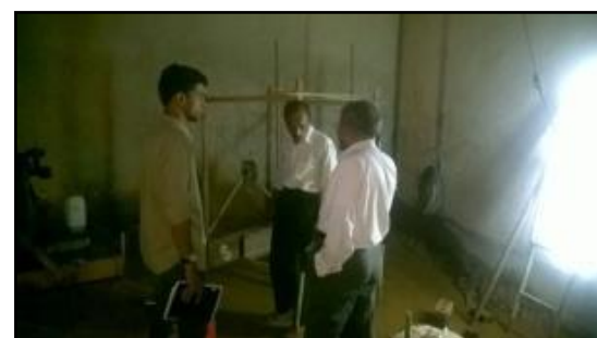
Fig.36 Discussion regarding the readings of load tests on piles with senior Engineer
