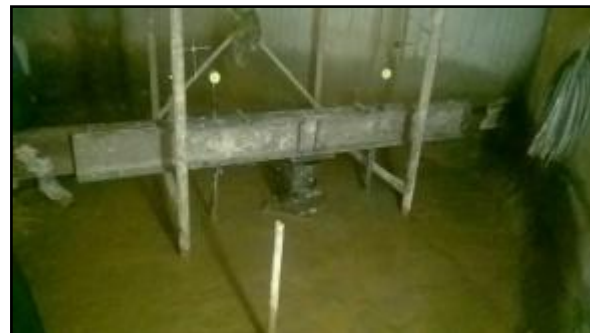
Fig.33 Setting of frame for dial gauges for load tests on piles
