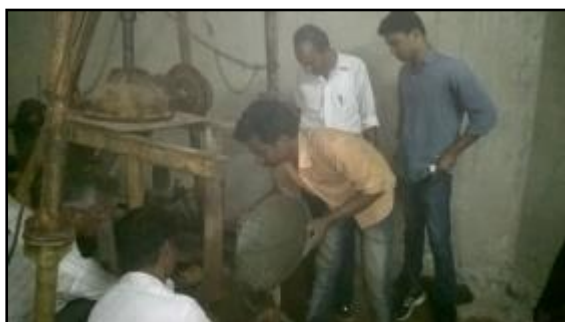
Fig.19 Concreting the bore hole
