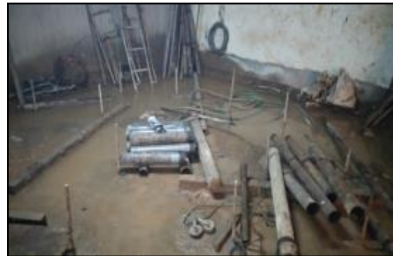
Fig.20 Removal of casing at each interval during the concreting work is in progress
