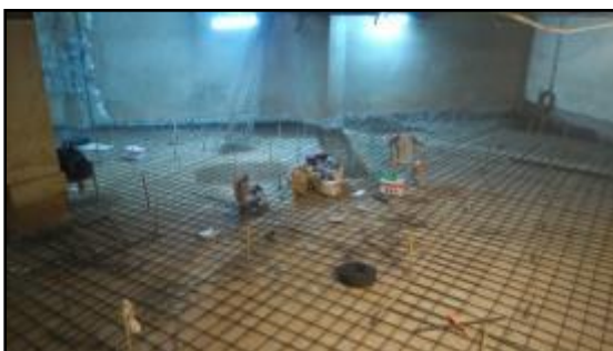
Fig.25 Laying of bottom steel
