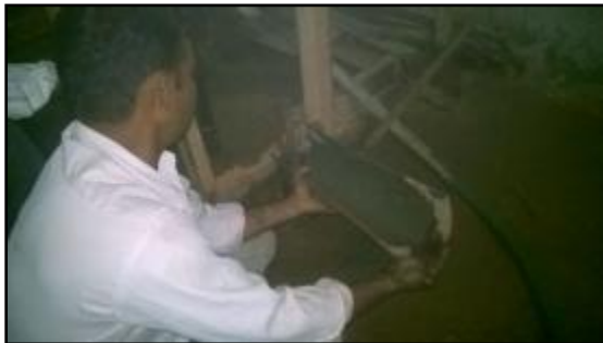
Fig.17 Placing the funnel for pouring of concrete
