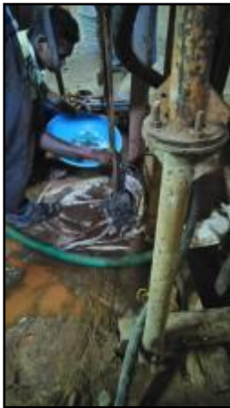
Fig.10 Putting the Lokfix (Grout) in the connecting pipe to connect the bars
